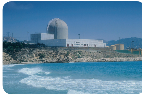
Central nuclear Vandellós II.
