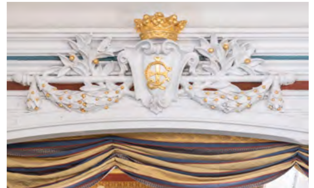
Crest with marquis crown and the initials of José Elduayen in the keystone of the arch over the main staircase.
