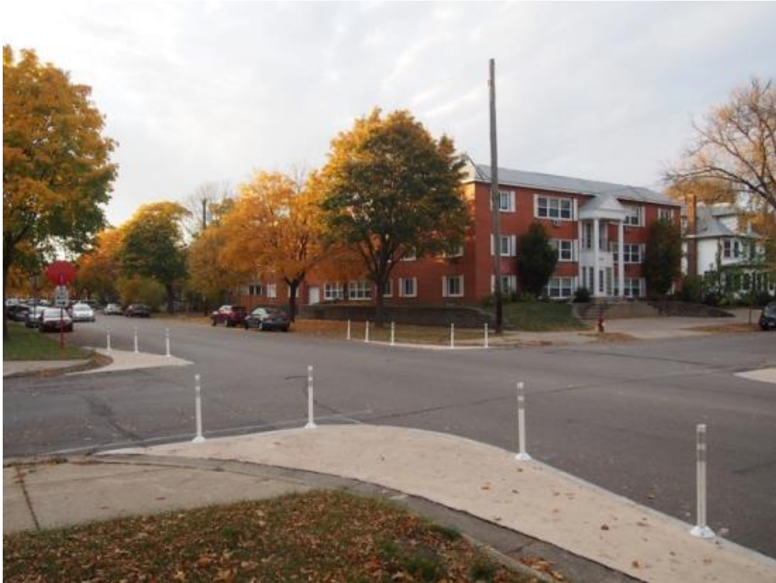
Paint and Flexposts (quick build)
