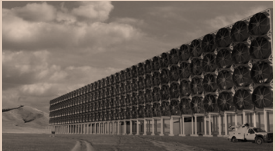
Design of Carbon Engineering air contactor (that could capture about a million tons of CO 2 per year)
