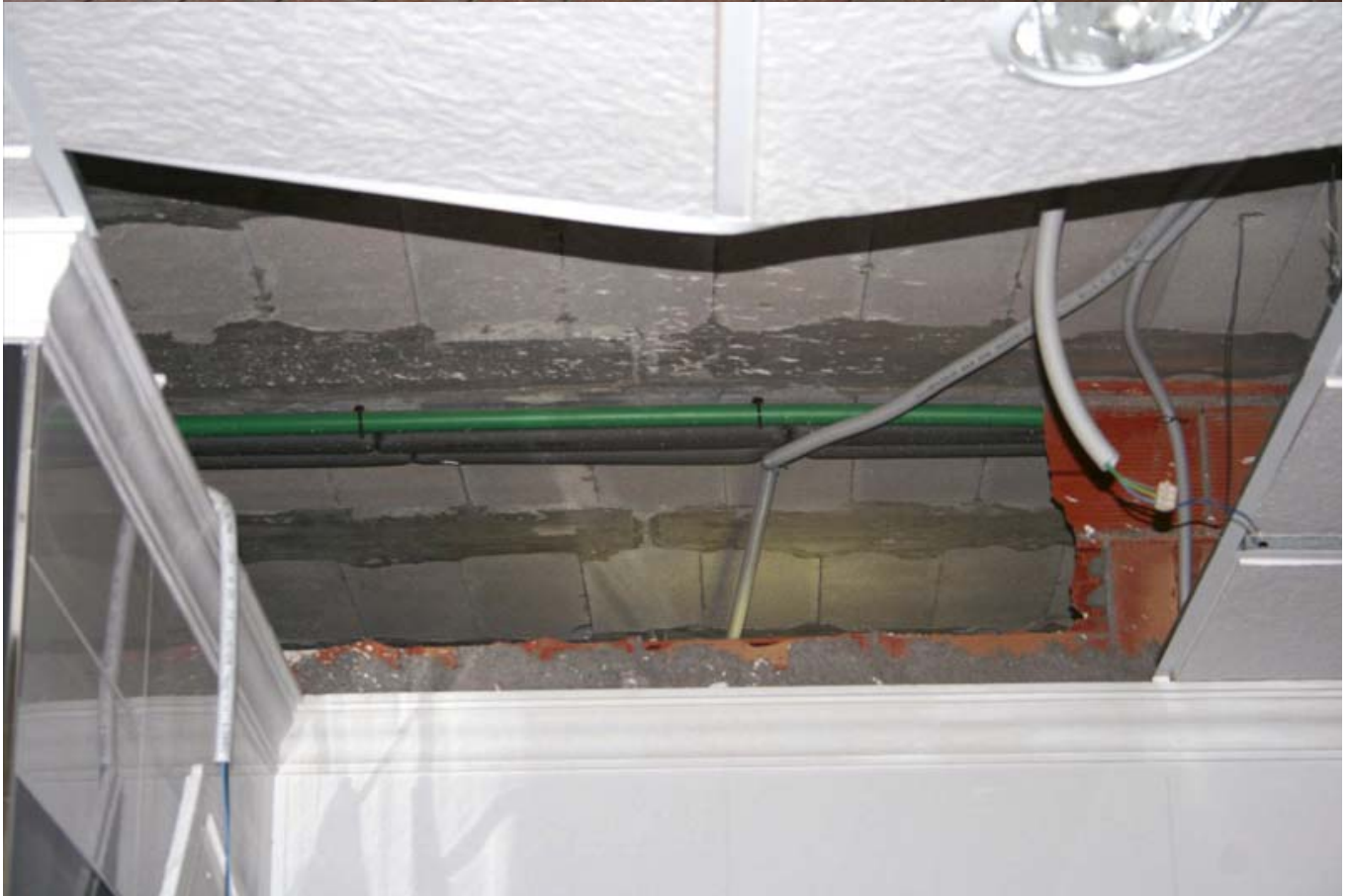
Figure 9. Petrol station damage caused by overpressure blast wave. Source (4) : Authors.
