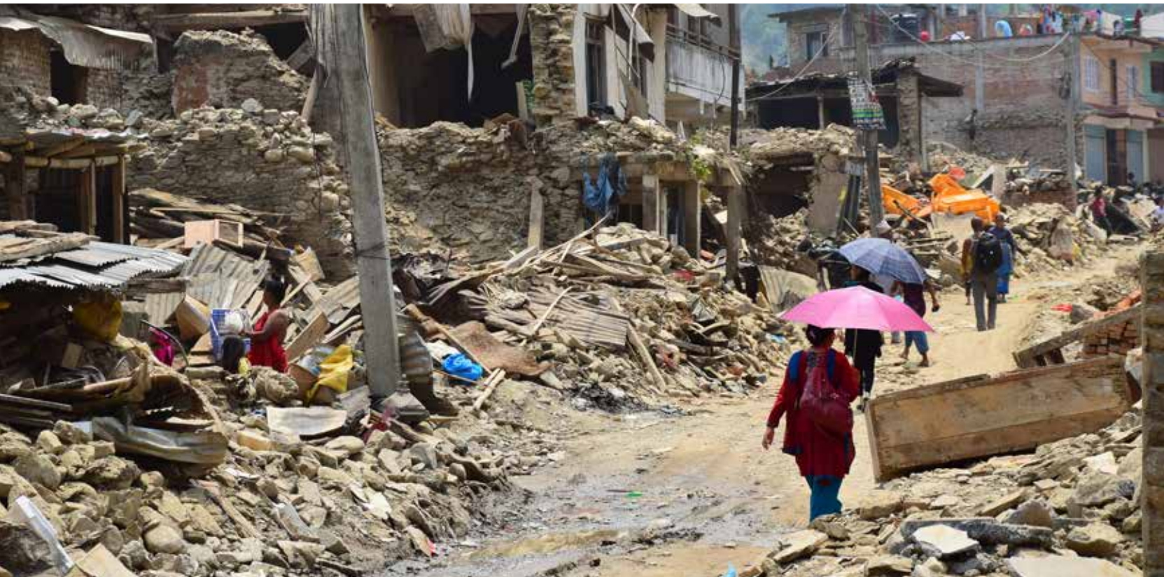
Sipaghat bazar, Kavreplanchok, Nepal after an earthquake.
