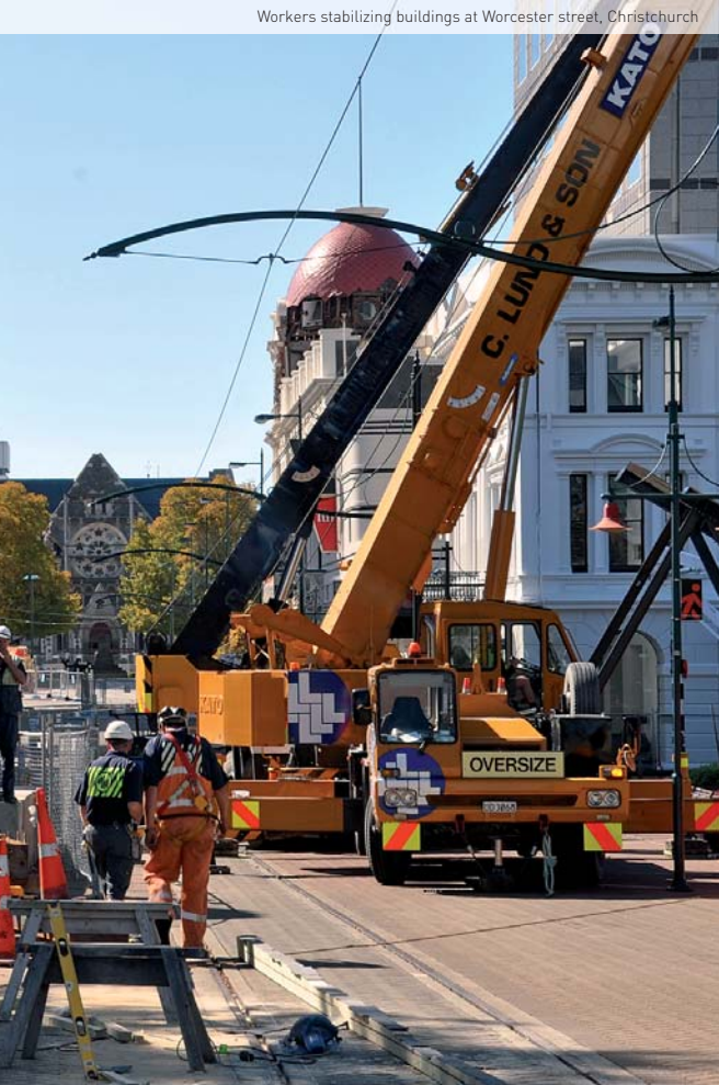
Workers stabilizing buildings at Worcester street, Christchurch
