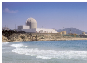
Central Nuclear Vandellós II
