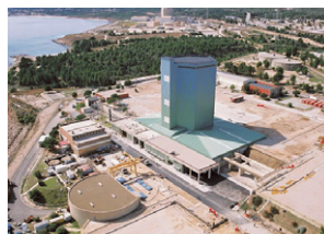
Central Nuclear Vandellós I
