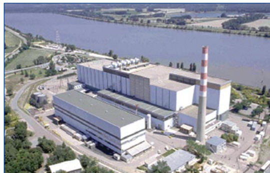
Reactor Phénix, Francia
