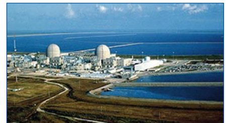
Central nuclear de South Texas (EEUU)
