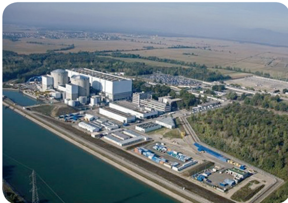
Central de Fessenheim (© EDF).
