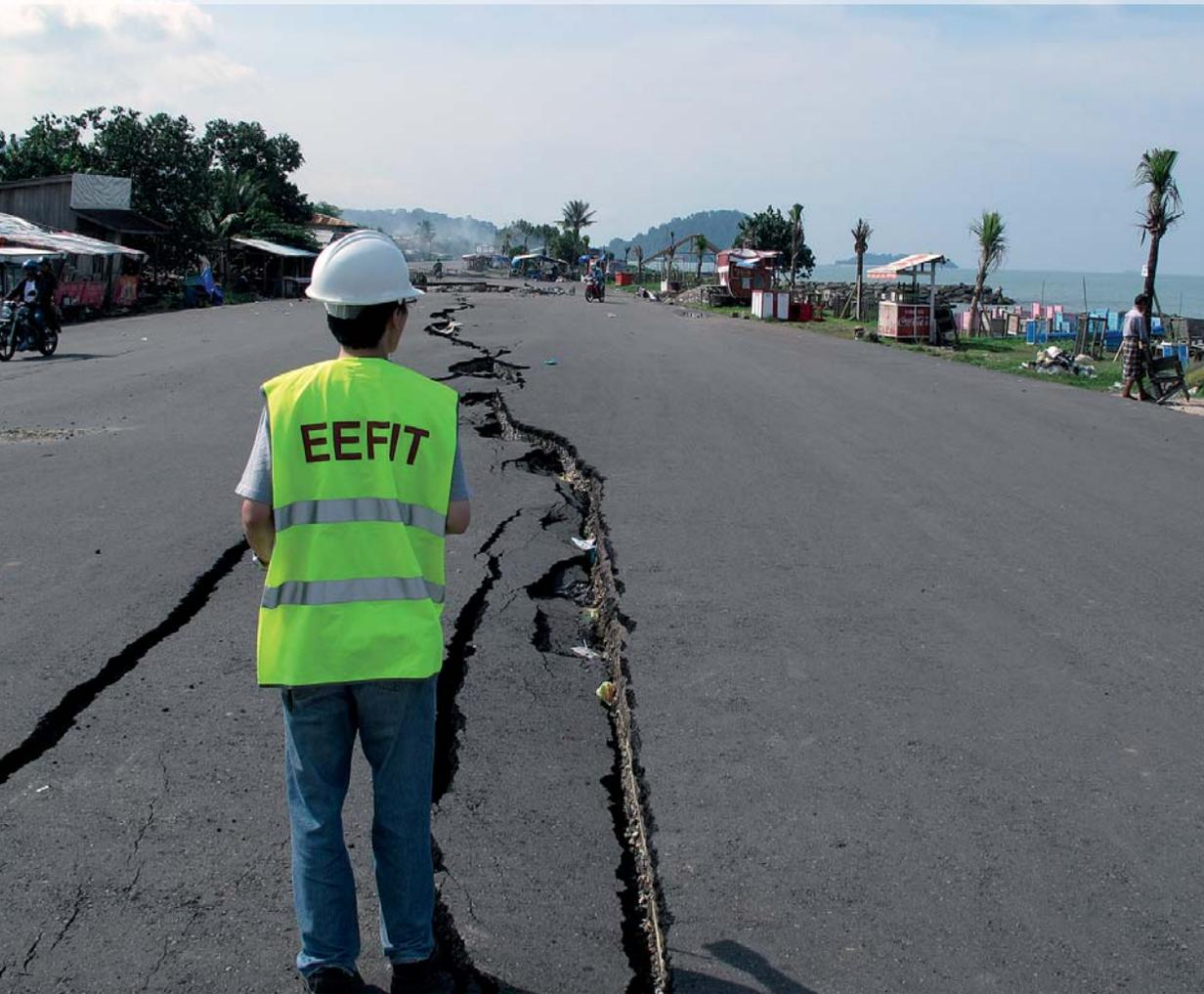
**Liquefaction is where the soil has essentially become like water and loses its strength causing structures to sink and topple over. There was a vast amount of liquefaction in both the Kocaeli earthquake in Turkey and Christchurch, New Zealand**
