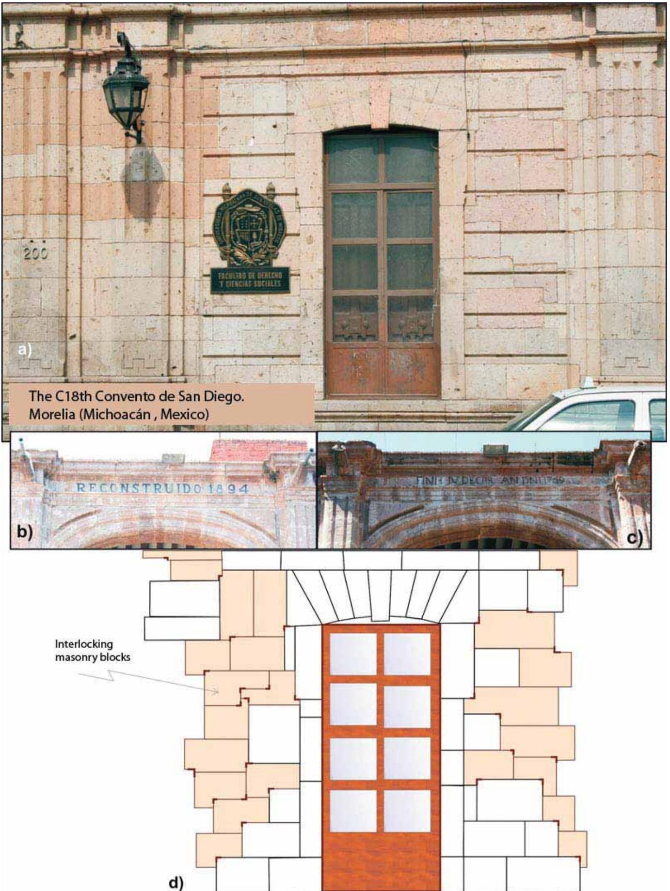
Figure 3. a) Detail of the 1884 reconstruction of the main front of the old Convento de San Diego (Morelia, México), with application of earthquake-resistant building techniques; (b) the reconstruction dates from the end of the nineteenth century (1895); (c) state after the great earthquake of Pátzcuaro (1856), which shook the towns of Pátzcuaro and Morelia. The main front reconstruction shows systematic use of interlocking masonry blocks (d).
