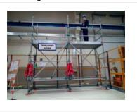
A training station prepared for explanation of the use of harnesses and ladders/stairs on site. Stress is laid on the scaffold identification tag number and prevention of falls from height in scaffold working.
