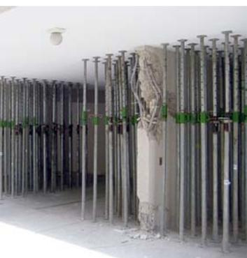
**Figure 9. Partial collapse of shear walls**
